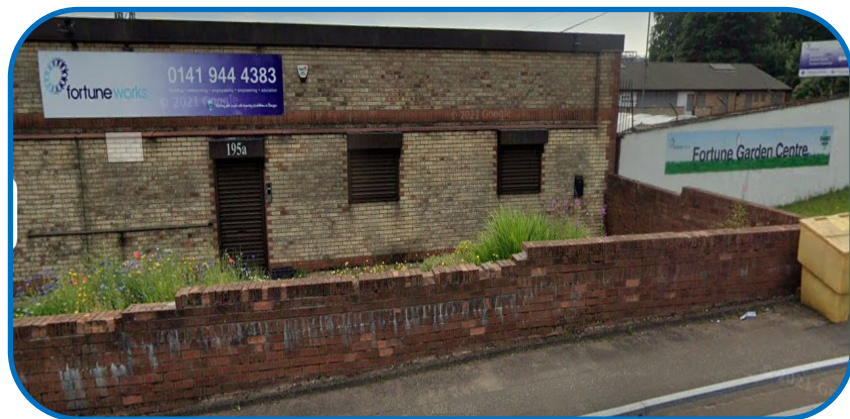
Enable Glasgow—Fortune Works
