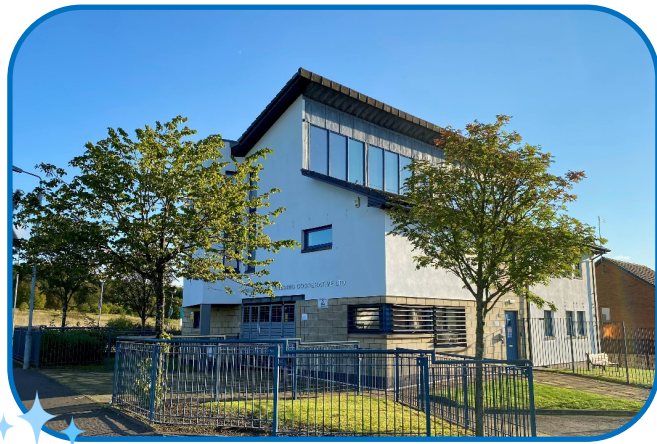
Glasgow – Drumchapel Housing Co-operative
