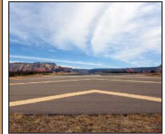
Runway 3 Threshold (Northeast)
