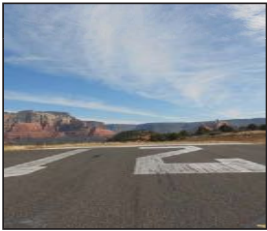
Runway 21 Threshold (Northeast)
