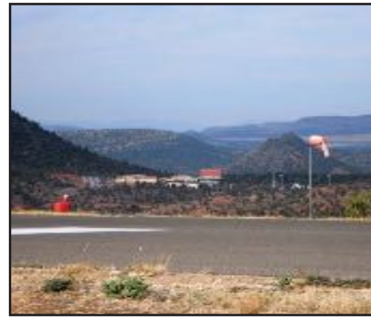
Wind Cone and REIL (Runway 3 Threshold)
