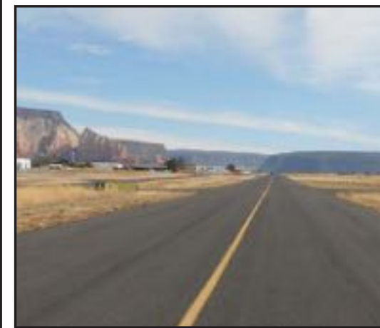
Taxiway A (Northeast)
