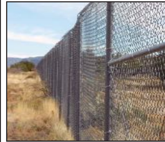
Perimeter Security Fencing
