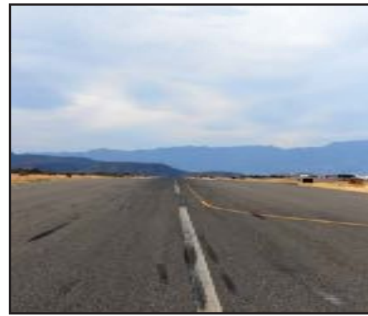
Runway 21 Threshold (Southwest)
