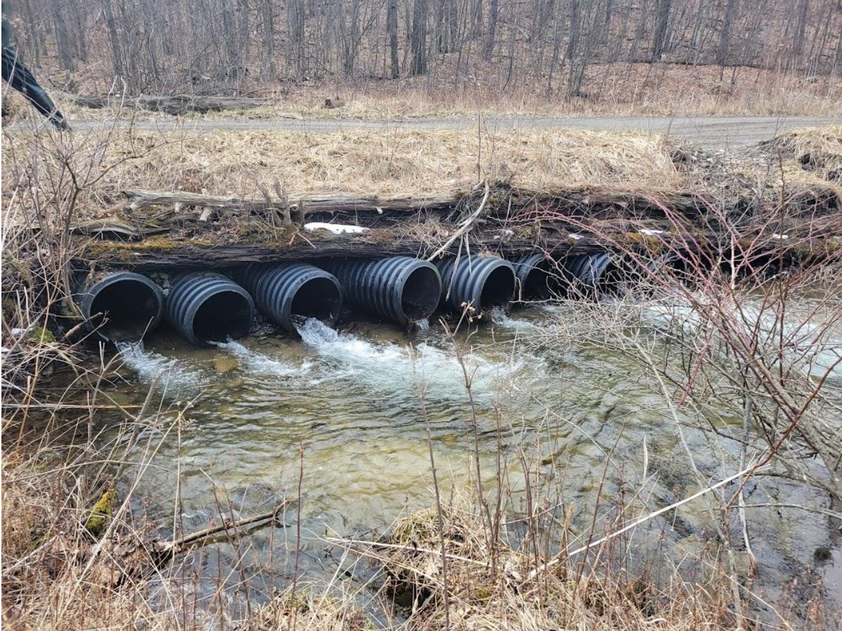
Figure 5a. Outlet of crossing with multiple pipes on Trim Root Run.
