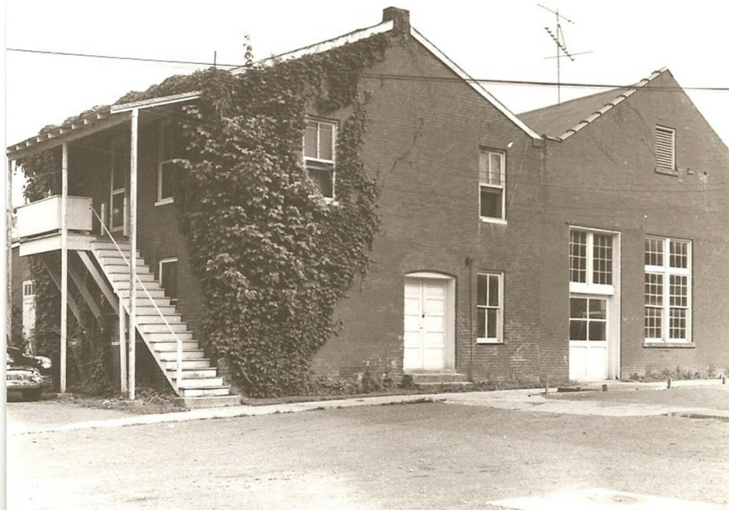
1903-1905. Heating Plant for steam, heat also ran the dynamo for the campus lighting system.
