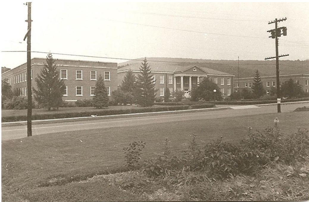
Dr. Krause secured P. W. A. (Public Works Administration) funds for the construction of the Elementary School for the Deaf (Primary Building) in 1937-38 at a cost of $290,000. Also constructed during this period of time were the Cannery in 1936 and the Laundry in 1937.
