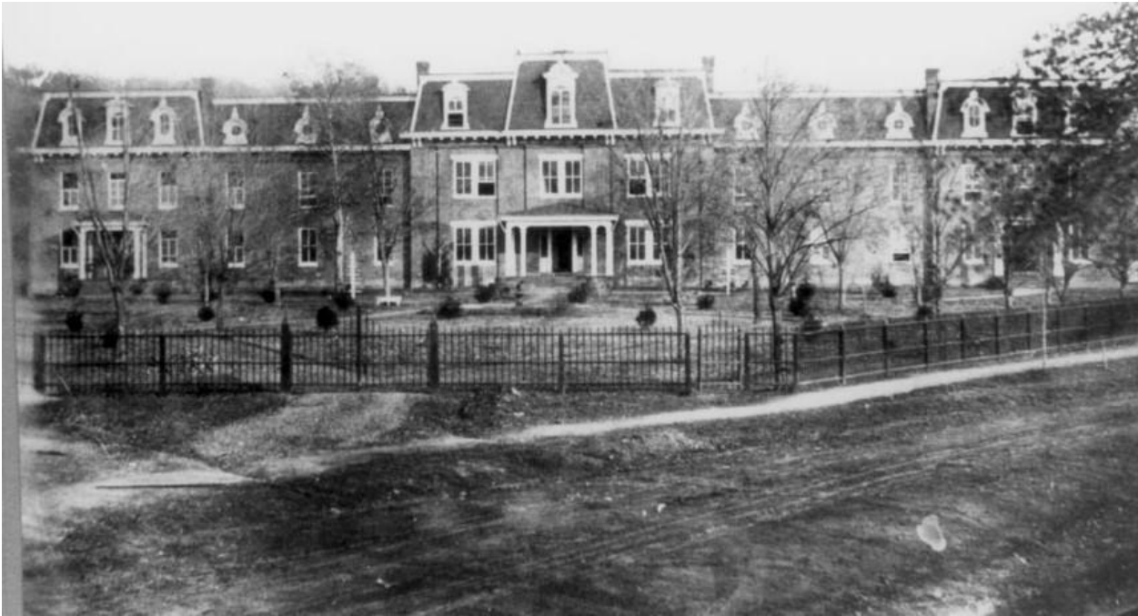
Front of Main Building following the addition of north and south wings and third floor. (source: http://www.historichampshire.org )
