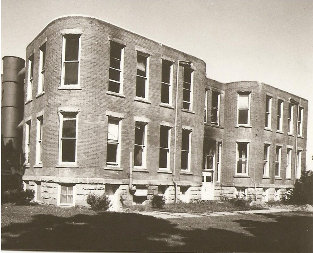
The smoke-stained brick shell and a blackened interior is all that remained of Rucker Hall following the fire.
