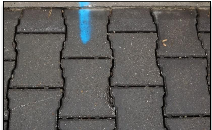
Photo 2 – PaveDrain following maintenance
