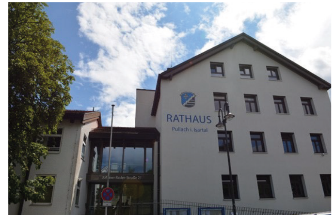
Pullach Town Hall heated by deep geothermal
