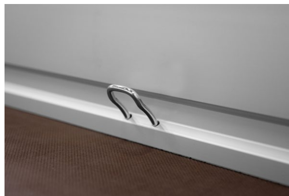
Recessed lashing eyelets
