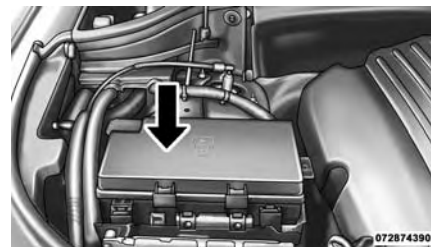
Power Distribution Center
