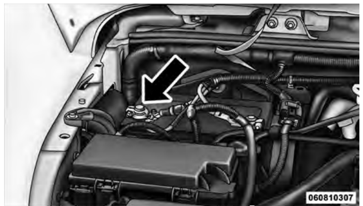
Positive Battery Post
