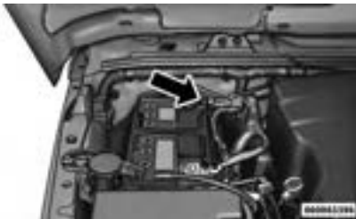
Positive Battery Post
