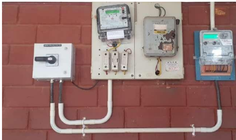
Solar inverter and other control devices
