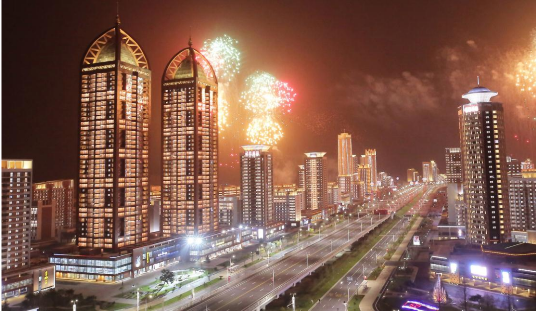
Hwasong Street completed in April 2023
