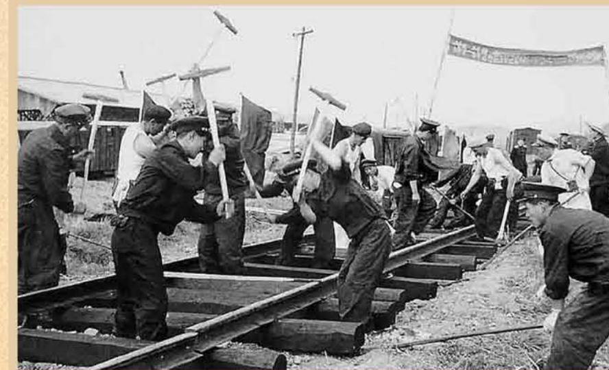
Railway workers laid in only 75 days 80km of standard-gauge railway lines between Haeju and Hasong.
