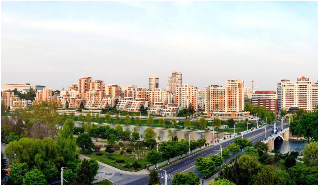
Panoramic view of the Pothong Riverside Terraced Houses District
