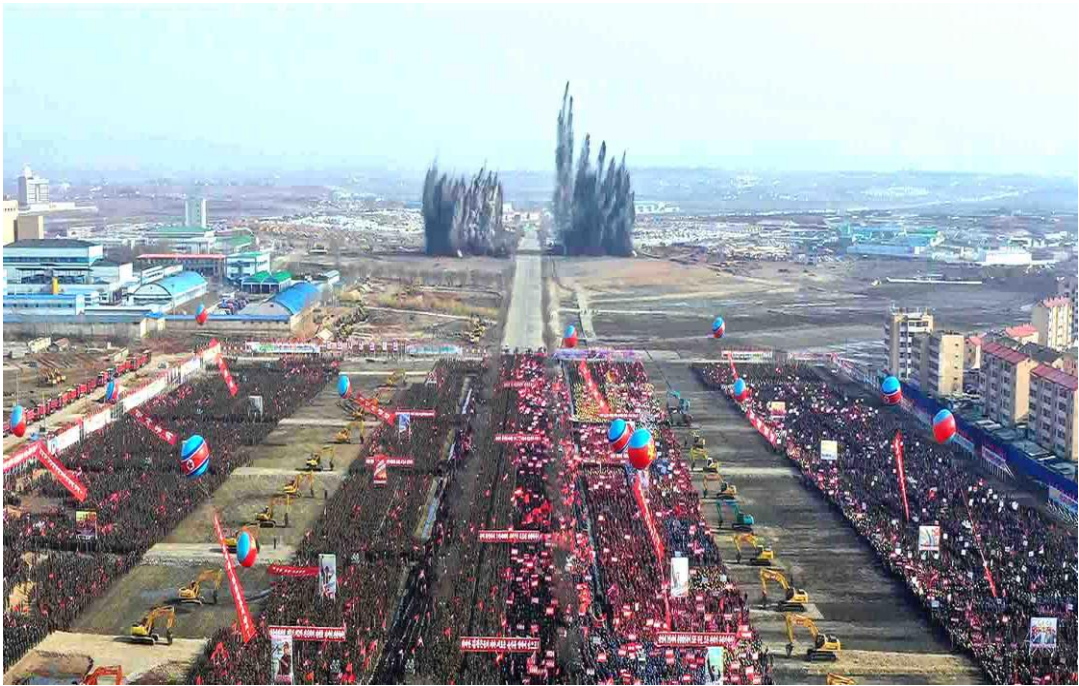
Groundbreaking ceremony held in March 2021 for building 10 000 flats in the Songsin and Songhwa area of Pyongyang
