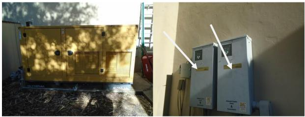
All of the electrical boxes for the generator do not have dead front panels installed.
