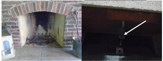
At the time of inspection the fireplace chimney flue was covered with creosote. Damper is operable. <u>Recommend having the flue cleaned and re-evaluated before</u> <u>operating the fireplace.</u>
