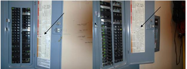
Various circuits within all of the sub panels in the upstairs laundry room were mis-identified, or the labels were illegible. Several areas of the legend have been covered over and re-labeled. They should be properly labeled for safety reasons, and so that the appropriate load calculations and breaker sizes can be determined.
