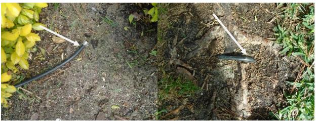
Large cut electrical line buried on the right side of the front yard. At the time of inspection the line was not live. (Safety hazard).
