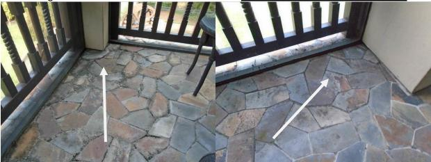
Portions of the rear balcony floor appear to collect water. The floor and the ceilings below were tested with moisture detecting and infrared equipment and tested dry. Possible hidden damage below the floor. <u>Recommend monitoring these areas.</u>
