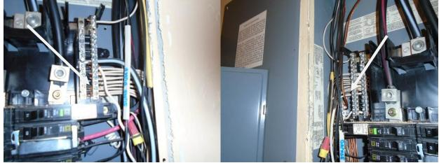
One or more neutral wires are incorrectly connected under a single screw on the grounding or neutral bus bar at the interior sub panels and should be serviced. Unless the manufacturer states otherwise, bus bars are only designed for one conductor per terminating screw.
