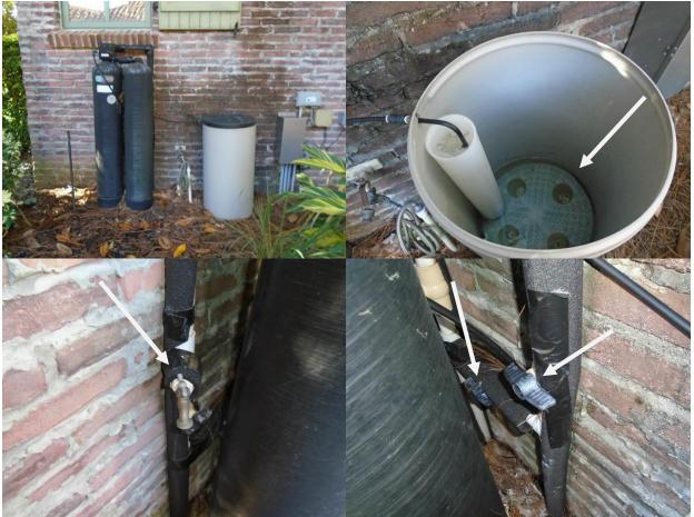
Water softener does not operate. The tank is empty and all valves have been turned off. Recommend further evaluation by a qualified contractor.
