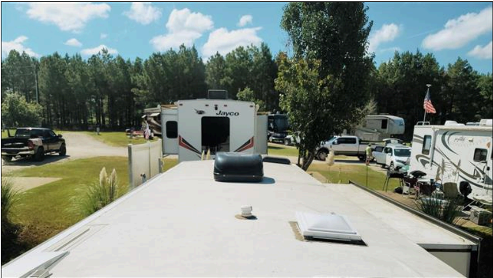
View of roof from rear to front
