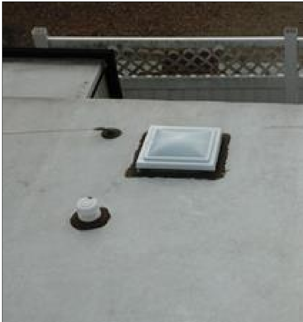
Overview of center bathroom skylight
