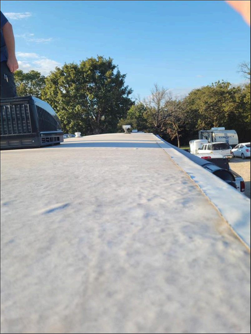
Overview of Roof - from back to front curbside
