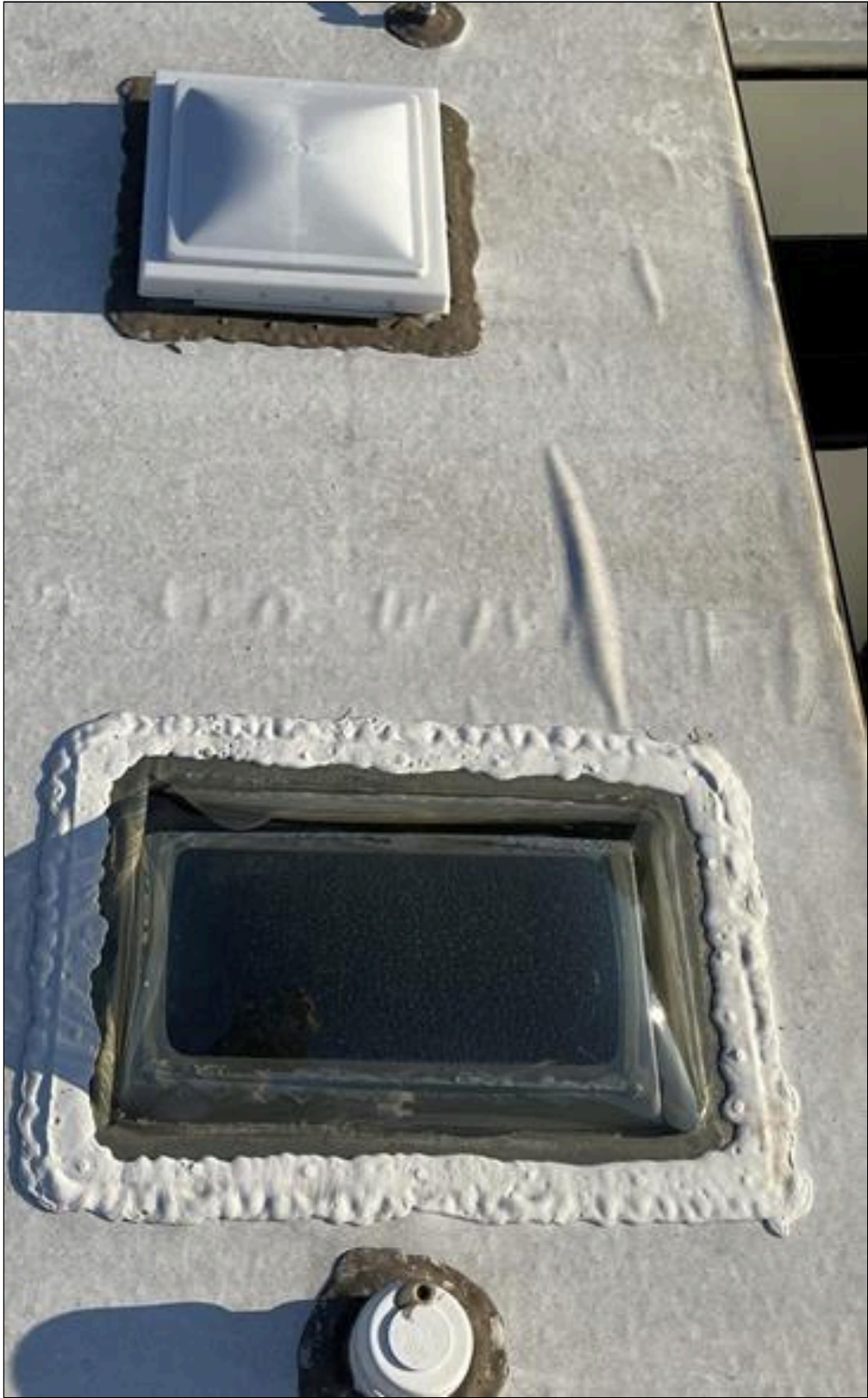
view of vents covers on roof
