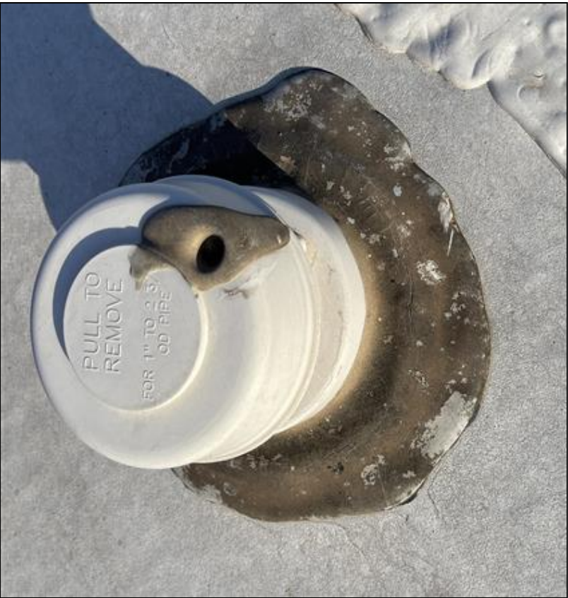
close up view of plumbing vent
