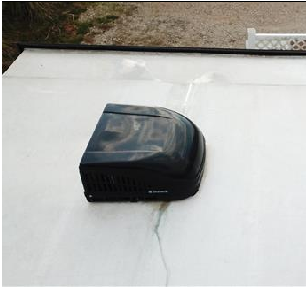
curbside view of A/C shroud
