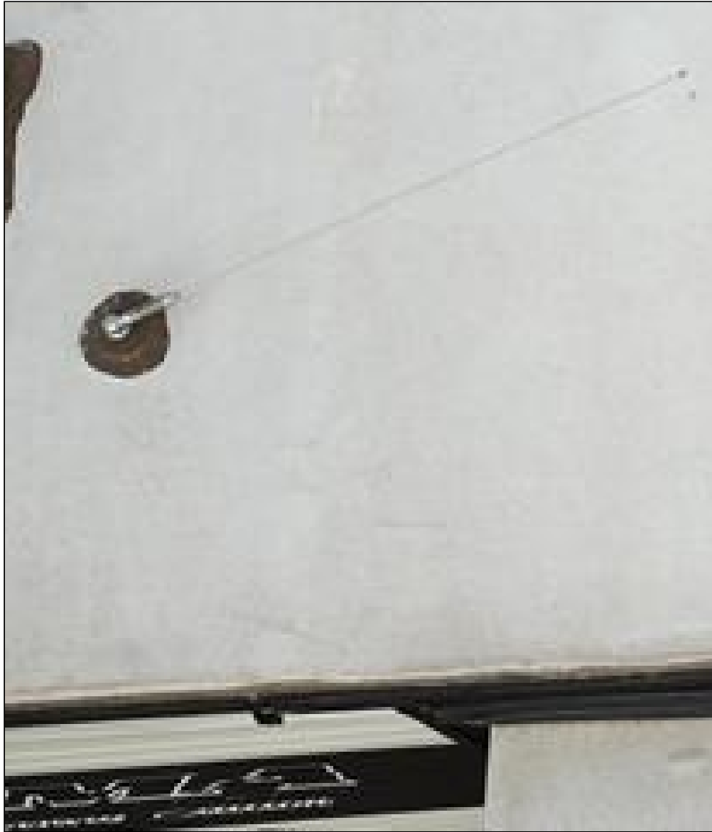
Radio Antenna top view
