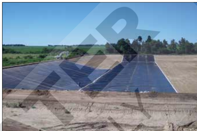
Waste Lagoon Liner
