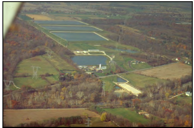
Del-Co Water Headquarters on S.R. 315, Liberty Township
