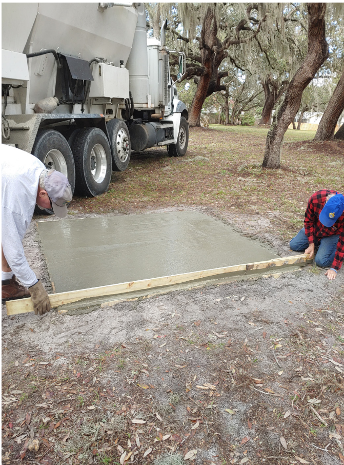
Danny Elliott and Danny McConnell pour cement in the form for the spiritual table.
