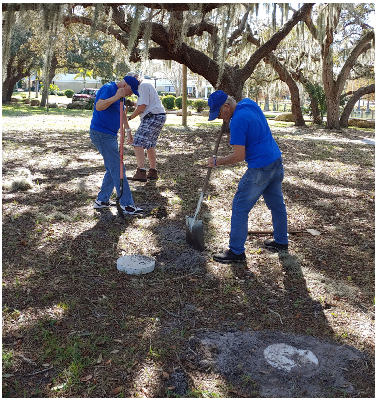
L-R: Bill Bannon, Danny Elliott, and Danny McConnell begin placing the cement circles where they belong in the ground for the rosary.
