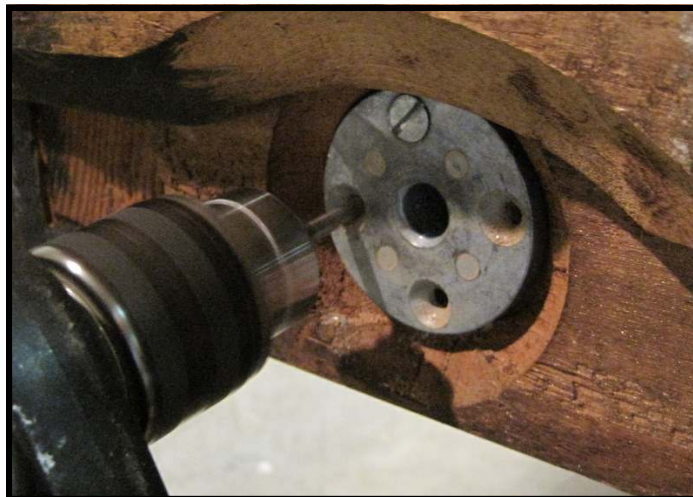
New socket being installed.
