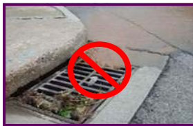
Grass clippings, leaves, and other vegetation placed in the streets is washed into storm inlet grates, which can block pipes, and causes an increase in the nitrate levels in the Chesapeake Bay.
