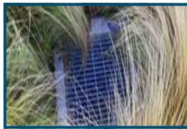
Above photos show rock pile, overgrown weeds, and flower bed blocking roadside swale inlets.
