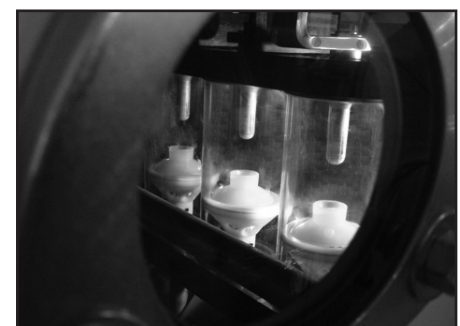
▲ Load break switch visible break.
