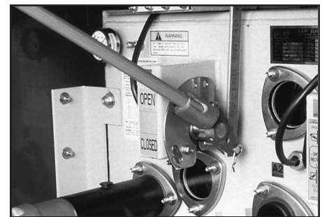
▲ Load break operating handle.
