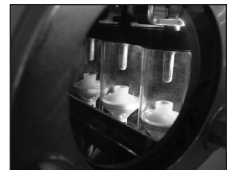
▲ Load break switch visible break.
