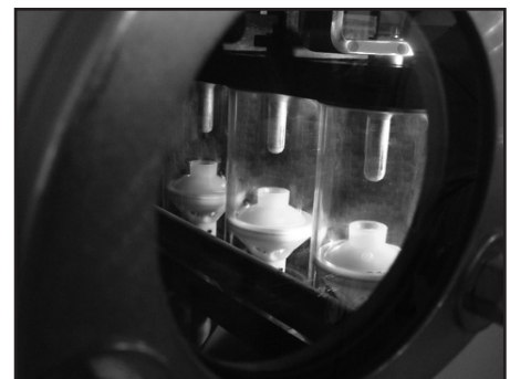
▲ Load break switch visible break
