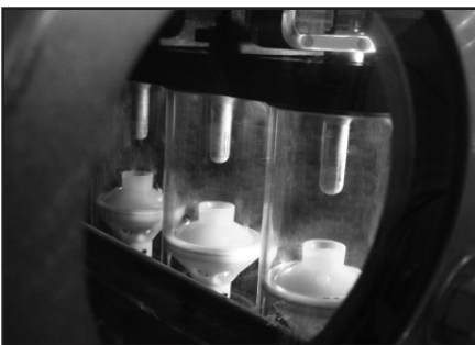
▲ Three phase visible position of contacts.
