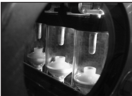
▲ Three phase visible position of contacts.
