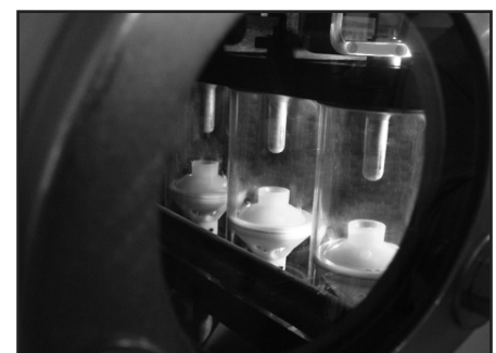
▲ Load break switch visible break.
