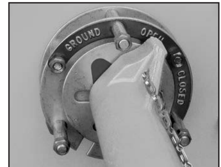
▲ Load break multi-position switch operator.
