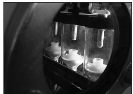
▲ Load break switch visible break.
