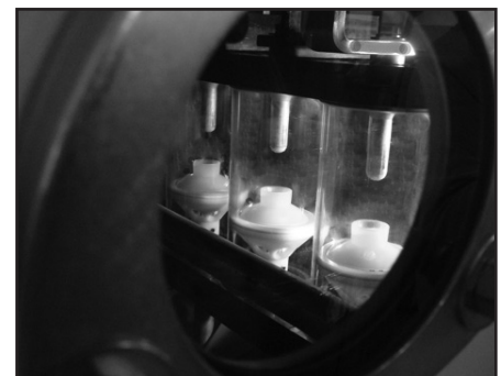
▲ Load break switch visible break.
