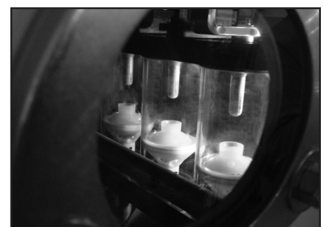
▲ Load break switch visible break.
