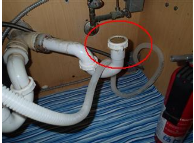
Inadequately capped drain under kitchen sink
