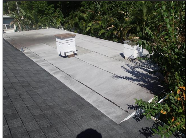
1.0 Item 2(Picture) Bee keeping boxes on flat roof
