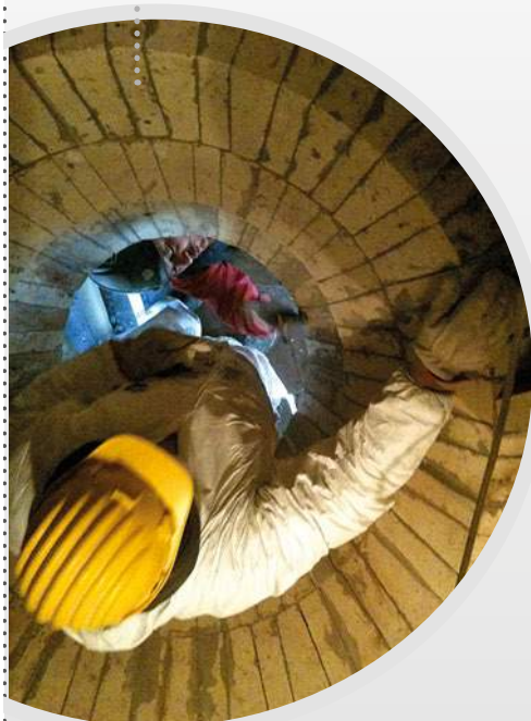
Cyclone – Bricks installation.
