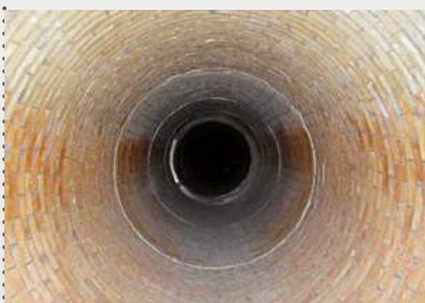
Tertiary air duct. Lined with fireclay bricks.
