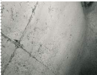
Smoke chamber. Low cement gunning application
