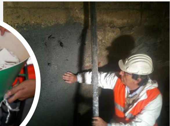
Shot Creting installation. Quality inspection
