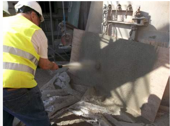
Gunning installation Tuning of the gunning machine
