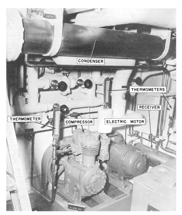
Figure 11-2.—High-pressure side of R-12 installation aboard ship.
