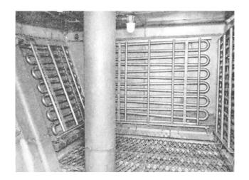
Figure 11-4.—Evaporator tubing.
