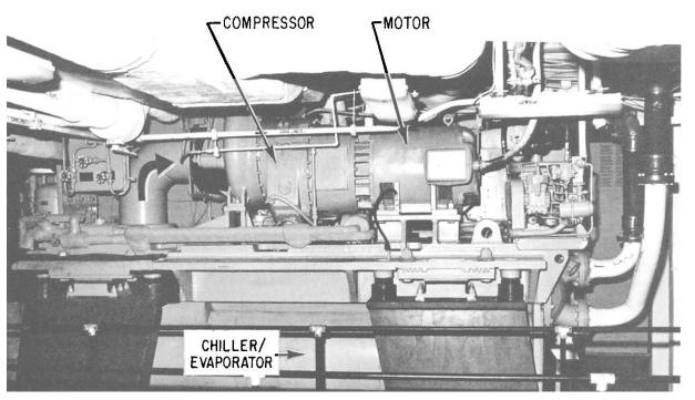
Figure 12-7.--R-114 centrifugal air-conditioning plant.
