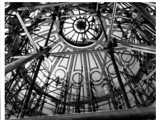
Tube & Clamp may be one of the most labor intensive scaffold systems, but the return on the time invested is nearly unlimited adaptability and access to even the most unique jobsite.
