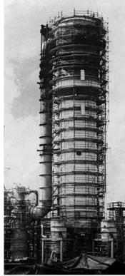
Left: Tube & Clamp encircles a tall stack. Right: Tube & Clamp provides access within a domed structure.
