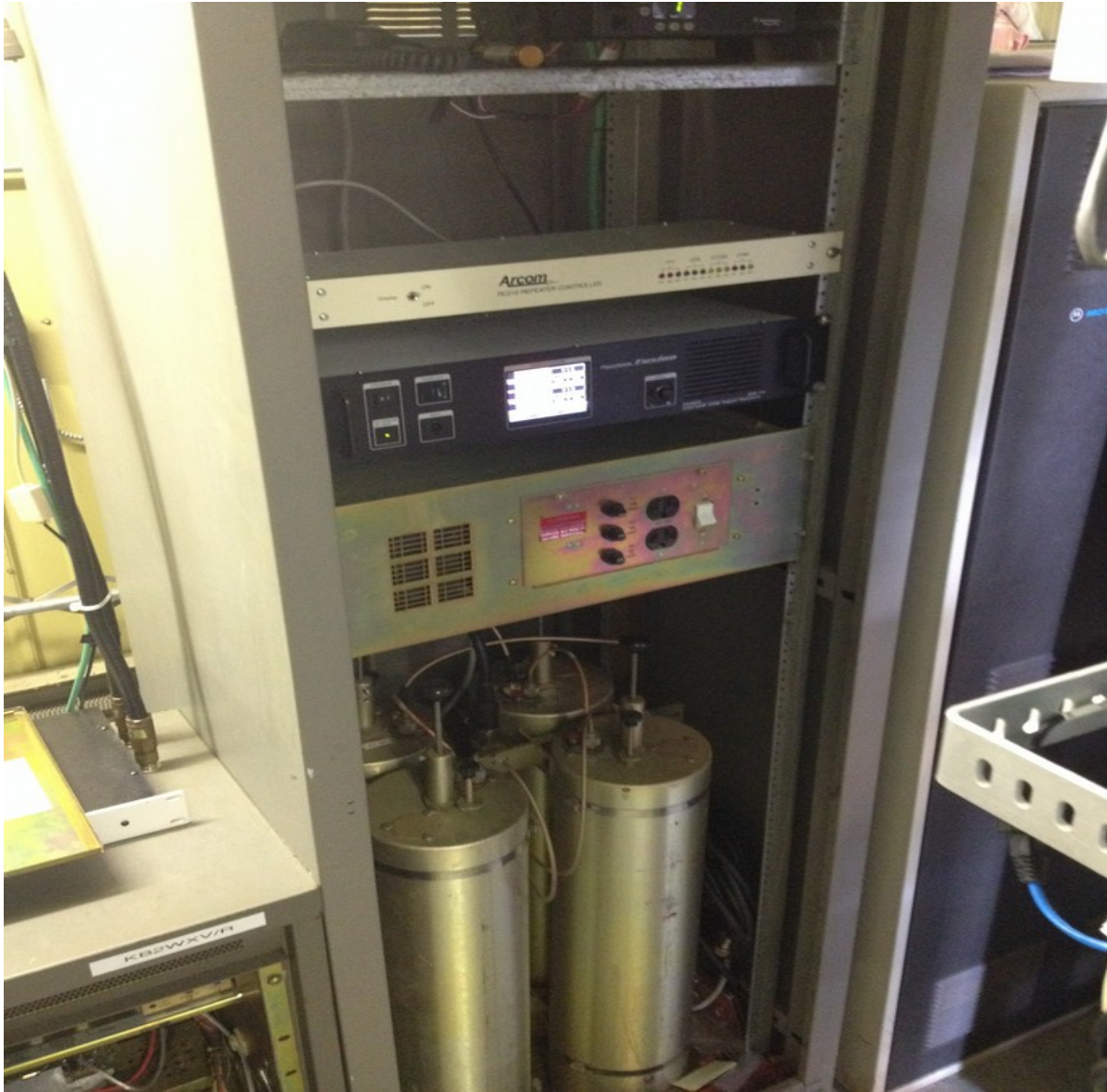
Cavity filters for the duplexer
