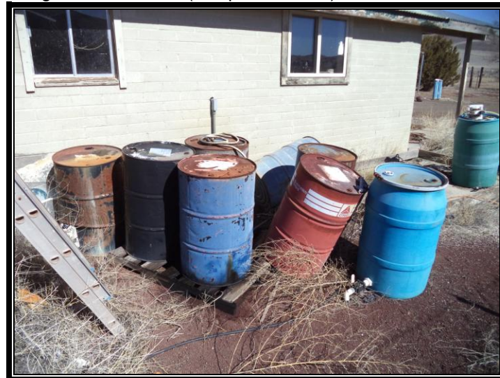
Photo No. 4: View of drums (mostly empty, some with waste oil) behind generator building.
