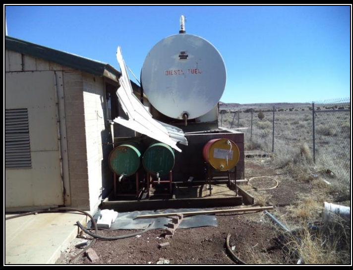
Photo No. 5: View of several drums on dispenser stands beside diesel fuel AST.
