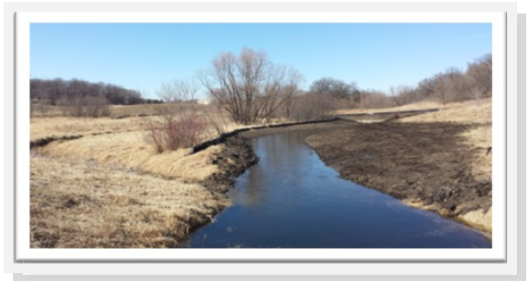
Early April CRWD PO 6 Project Enhancement | Looking north from HWY 55, addition of channel to reduce phosphorus load to Cedar (original stream to the left)
