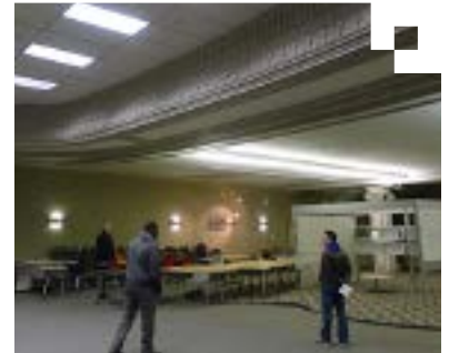
2018 view of dropped ceiling showing balcony front railing
