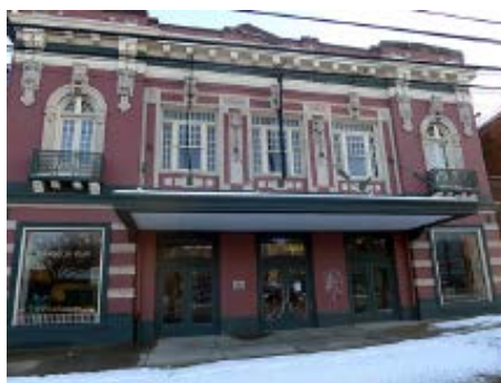
Current view of front—2018
