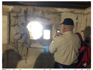
This hole was made by a 14 inch shell fired from the USS Nevada. The shell passed through the main gun port without hitting the gun. It did not explode but did pass through not only the rear wall of the gun port but passed through another corridor wall before burying itself in the ground behind the bunker. The concussion from the strike killed the entire gun crew.
