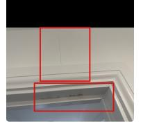
Similar To Previous Issue - Main Bathroom Door Needs Easing Suggested Assigned To: Carpenter / Decorator Amber item - ease bathroom door and make good movement cracks that had occurred from this
