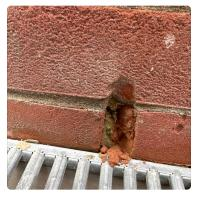
Damaged Brick Work To Front Of Garage Suggested Assigned To: Brick Layer / Surface Specialist Green item - replace / fix damaged brick
