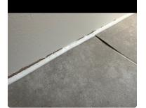
Perished Mastic And Lifting Amtico In Main Bathroom Suggested Assigned To: Mastic And Floor Layer Green item - sort flooring and refresh sealant
