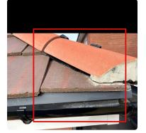
Loose Roof Tile Garden Side Of Garage Roof Suggested Assigned To: Roofer
