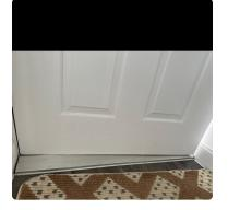
Ease Front Door - Scraping On Bottom Suggested Assigned To: Carpenter Amber item - door needs significant adjustment
