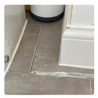
Loose Amtico Tile RHS of Toilet In Main Bathroom. Suggested Assigned To: Floor Layer Green item sort out lifting flooring
