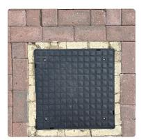
Another Drain Pot Cover With Cracked Pointing Surrounding It Suggested Assigned To: Groundworkers
