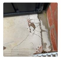
Driveway Floor Latexed For Some Reason (and Is Failing) Suggested Assigned To: Groundworker / Site / Floorer Amber item - latex is failing to garage floor all over
