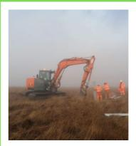
WE HAVE BEEN INSTALLING PEAT AND PLASTIC PILED DAMS USING LOW GROUND PRESSURE EXCAVATORS THAT WILL SERVE AS A NATURAL FLOOD MANAGEMENT TECHNIQUE. THE METHOD ALLOWS FLOOD WATER TO BE HELD **UPSTREAM AND RELEASED** SLOWLY, LOWERING THE CHANCE OF FLOODING IN DOWNSTREAM AREAS.
