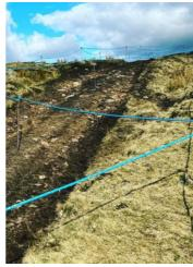
ONE OF OUR TEAMS HAS BEEN AT **SWELLANDS** INSTALLING **DETERRENT MEASURES** ALONG THE NEW 2KM ACCESS TRACK PRIOR TO CONSTRUCTION WORKS COMMENCING. WE USED GPS SURVEYING EQUIPMENT TO MARK THE NEW ACCESS ROAD AND PASSING PLACES AND THEN INSTALLED 14MM OF BLUE NYLON ROPE IN A ZIG ZAG PATTERN RAISED 1M OFF THE GROUND TO HELP DETER NESTING BIRDS.
