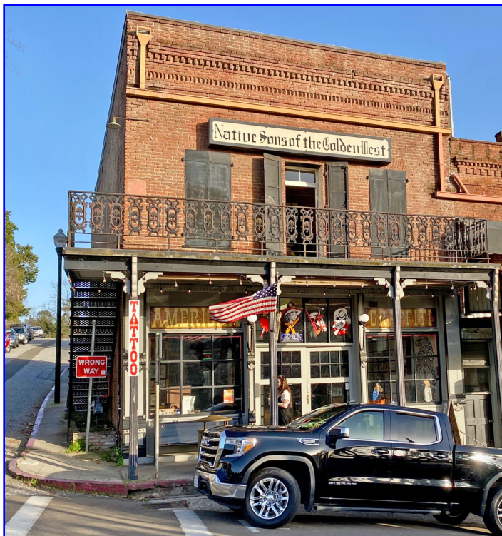
Auburn Parlor's historic hall.
