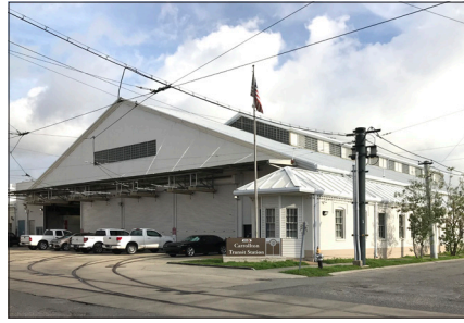
The City's streetcars are maintained at the Carrollton Transit Station.
