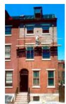
These qualities could be easily damaged by painting the brick, by raking out the joint with power tools, or repointing with a joint that is too wide. As seen here during the process of repointing, the visual character of this front wall is being dramatically changed from a wall where the bricks predominate, to a wall that is visually dominated by the mortar joints.
