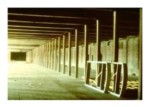
If features of the **structural system** are exposed, such as loadbearing brick walls, cast iron columns, roof trusses, posts and beams, vigas, or stone foundation walls, they may be important in defining the building's interior visual character.
