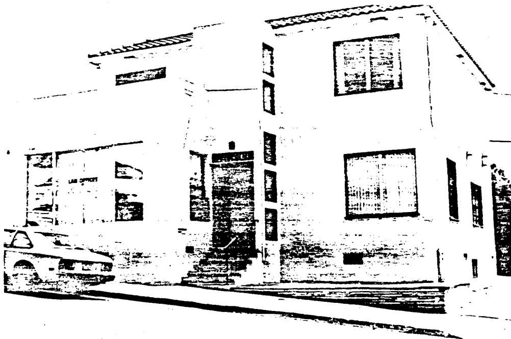
40 North Fir Street
