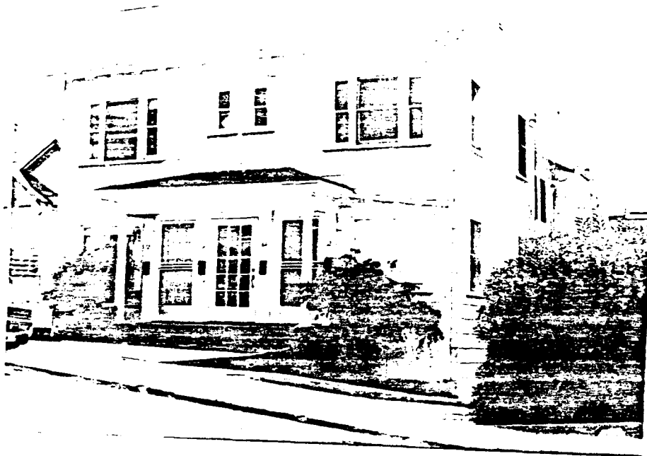
62-68 North Fir Street
