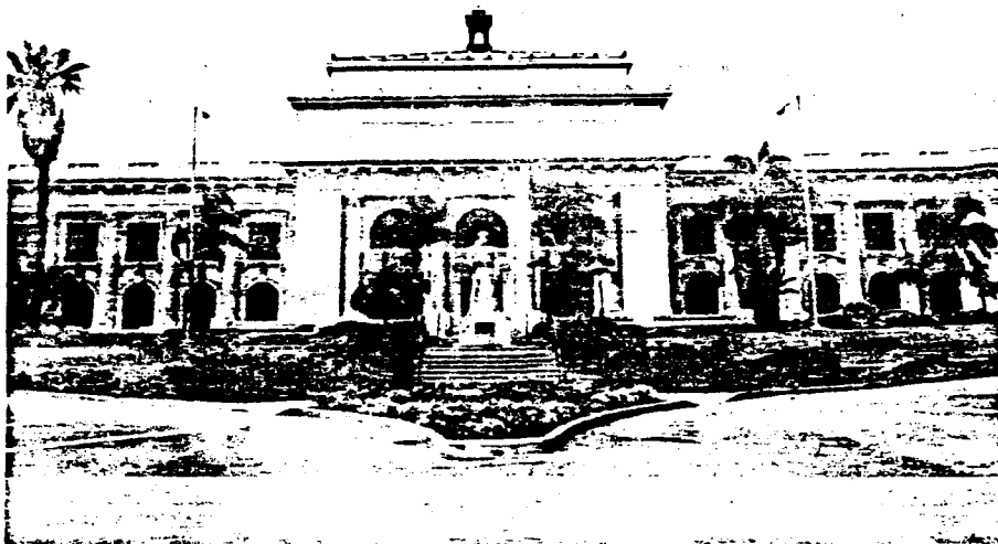
501-Poli Street Ventura County Courthouse
