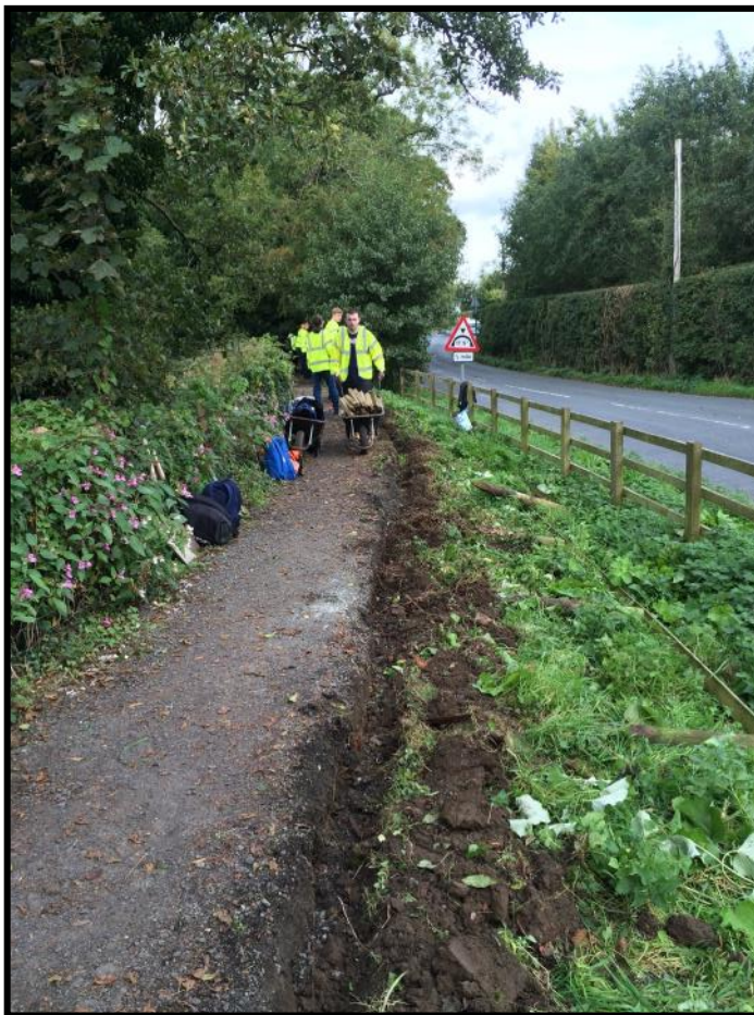
Above - Students replacing path edging on the Millenium Way which runs alongside the River Wyre.
