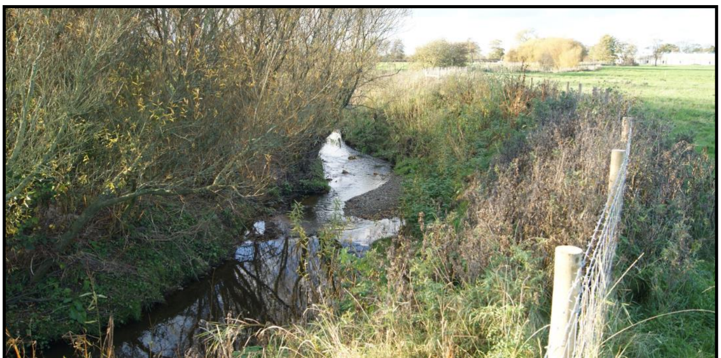
Above - The deposition of gravels and creation of a riffle around an area of bank restoration
