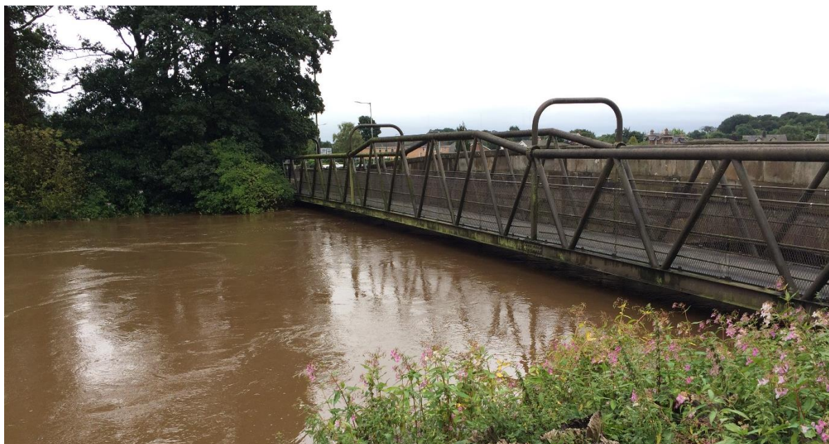
Figure 11 St Michaels road bridge, August 2016
