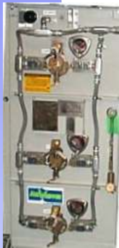
3 Phase loop switch configuration with transformer switch
