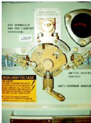
Switch Position Contacts
