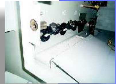
Bay-O-Net fusing and interlock
