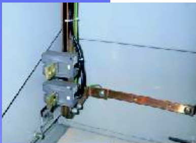
LV Grounding Connection
