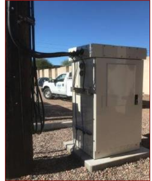
Rear View of Head End Node - Coax ingress via weather tight ports
