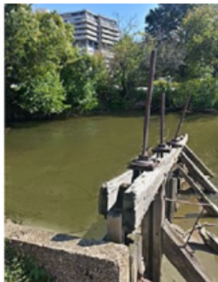
The C&O Canal terminus at milepost zero. The photo shows the remains of Waste Weir #1 , and where the gravity dam used to be. The "Watergate West" building is in the background.
