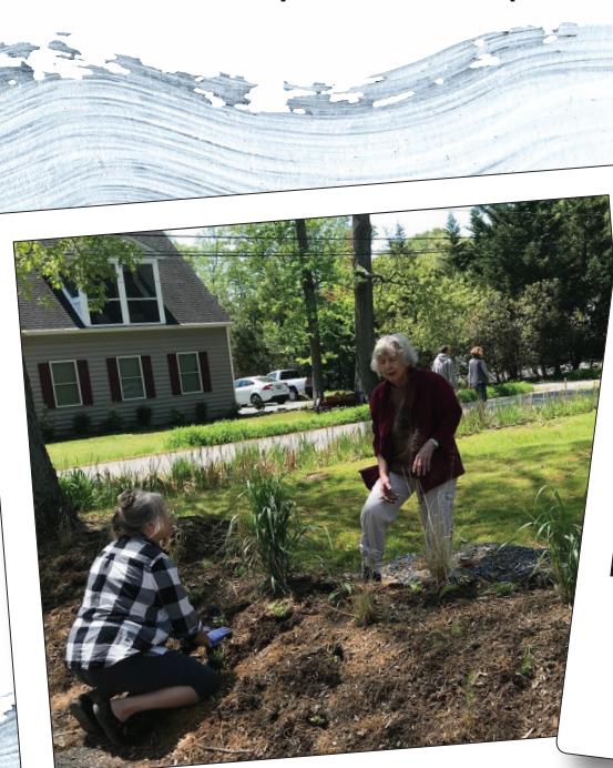
The new berm in our renovated parking lot got a major planting by volunteers to finish off the new parking lots project!
