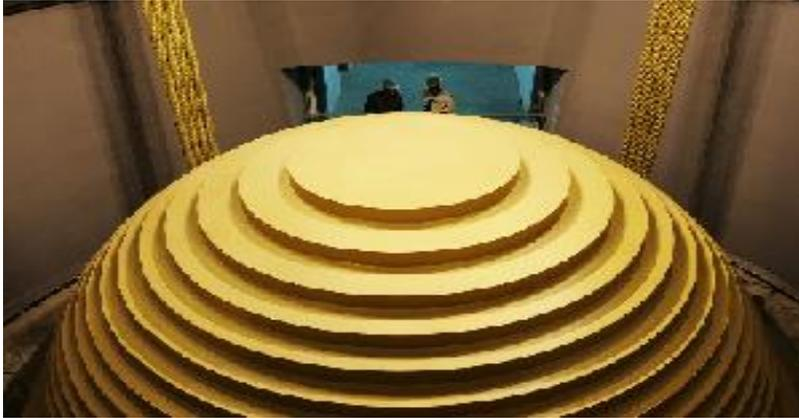
*A 660-ton spherical device called a tuned mass damper swings like a giant pendulum in the skyscraper's upper floors.*
