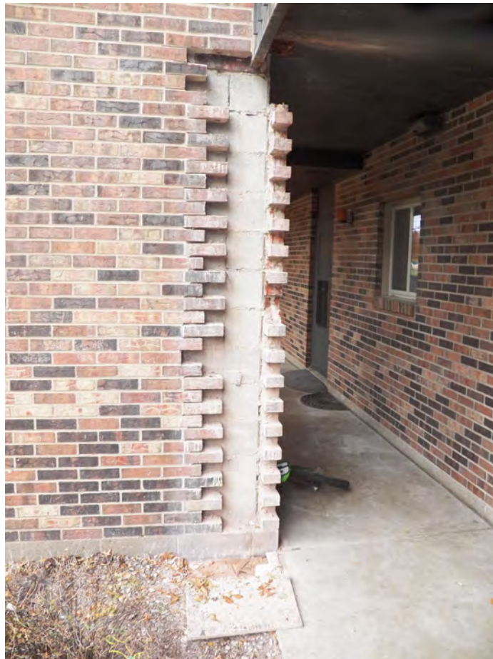
6. Partial brick demolition and foundation at Building A4.
