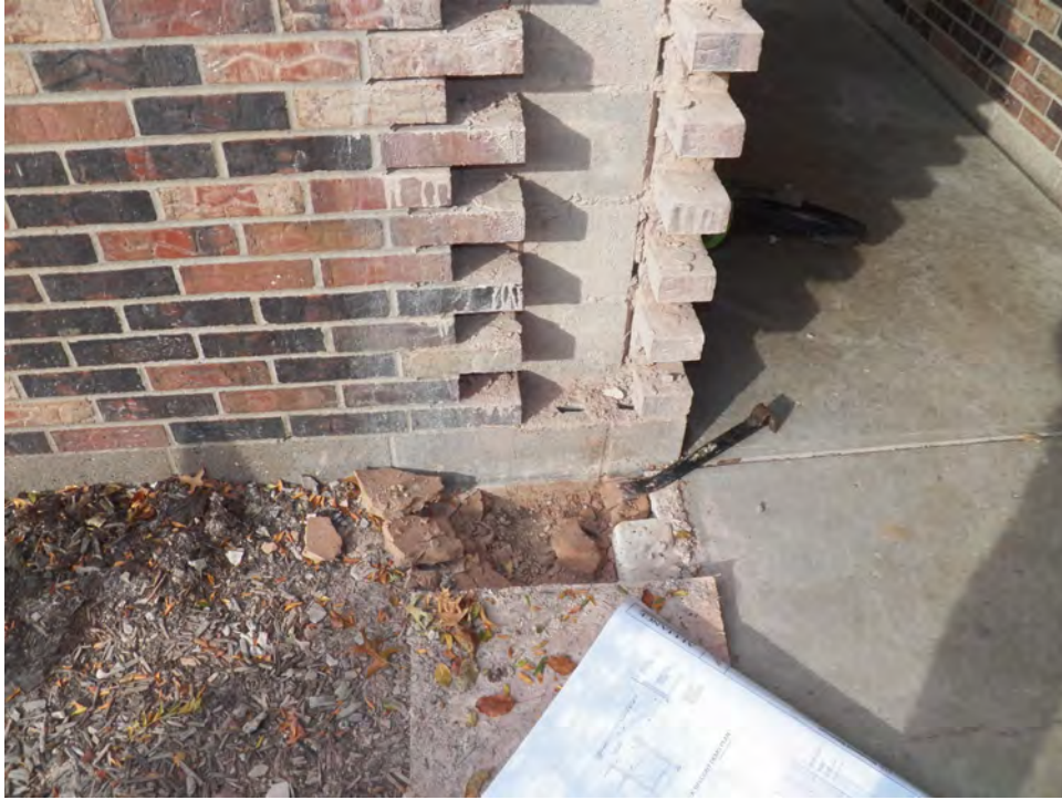
7. Partial brick demolition and foundation at Building A4.
